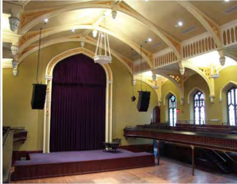
photos: left A dV-DOSC array covering the rear center balcony area. right KUDO for FOH, plus 112XT for side balcony coverage
