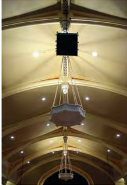
photos: left A dV-DOSC array covering the rear center balcony area. right KUDO for FOH, plus 112XT for side balcony coverage
